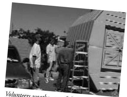
Volunteers weather-proofed an outside storage shed before the monsoon season.
